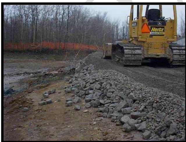
Figure 5: Roadway at Barker Chemical Site
