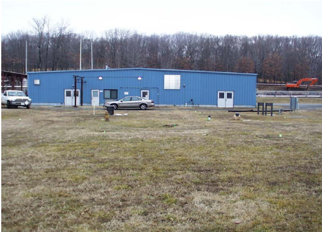
Figure 3-1B. Hog Out facility in Bldg 1419 (photo source: Carey Yates, IHDIV-NSWC)
