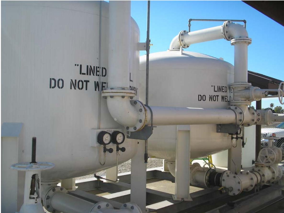
**Figure 12.** Face Piping and Well Connection – West Valley Water District
