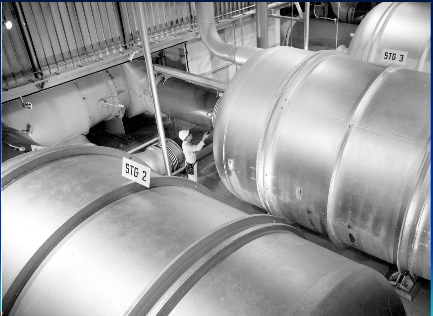
K-25 enrichment converters. Eventually there were five large enrichment buildings
