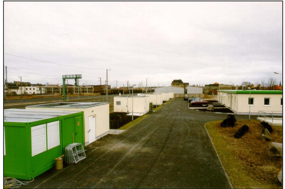
Figure 1: The SAFIRA test site with the five well shaft housings on the left-hand side and the on-site laboratory building on the right-hand side
