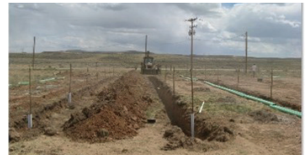
Figure 3. Tree Poles Planted in SGBR (Courtesy of Trihydro Corp.)
