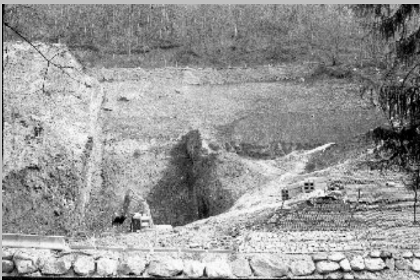
Figure 6.22: Nantieux landfill during remediation (Photograph courtesy of INERTEC)
