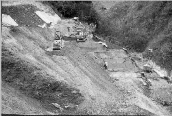
Figure 6.23: Nantieux landfill remediation operation nearing completion (Photograph courtesy of INERTEC)
