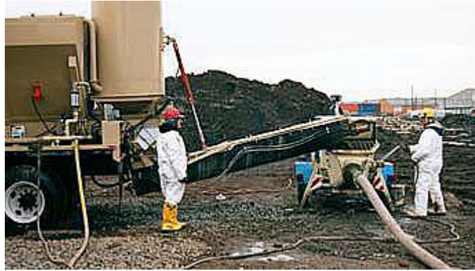
Figure 6.9: Mobile mixing plant to slurry pump by conveyor (Photograph courtesy of Keith Bradshaw)
