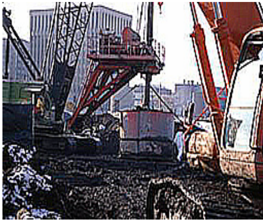
Figure 6.17: Large single auger (10ft diameter) with vapour extraction hood (and auger detail) (Photograph courtesy of Portland Cement Association)
