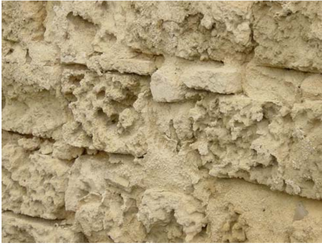
Figure 9.5: Surface decalcification of building stone, Bari, Italy. (Photograph courtesy of Brian Bone)
