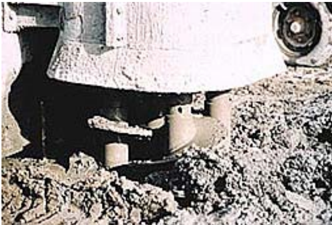
Figure 6.16: A quadruple auger penetrating contaminated soil (Photograph courtesy of Bachy Soletanche)
