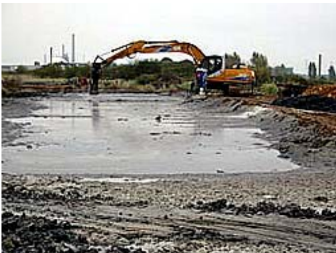
Figure 6.15: In-situ mixer treating a tar lagoon (Photograph courtesy of Colin Hills)
