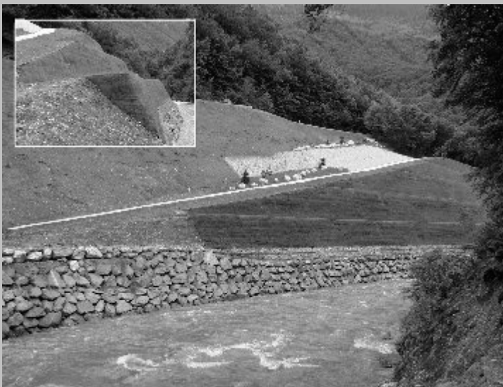
Figure 6.24: The completed project at Nantieux (Photograph courtesy of INERTEC)
