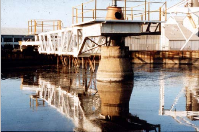
Figure 7.3: Lagoon for blending and dewatering wastes at Thurrock (photograph courtesy of Colin Hills).
