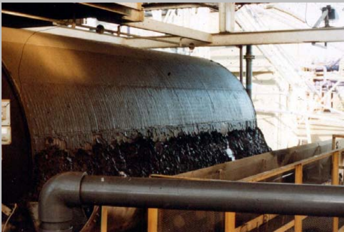
Figure 7.4: Vacuum filtration and production of filter cake at Thurrock (photograph courtesy of Colin Hills).
