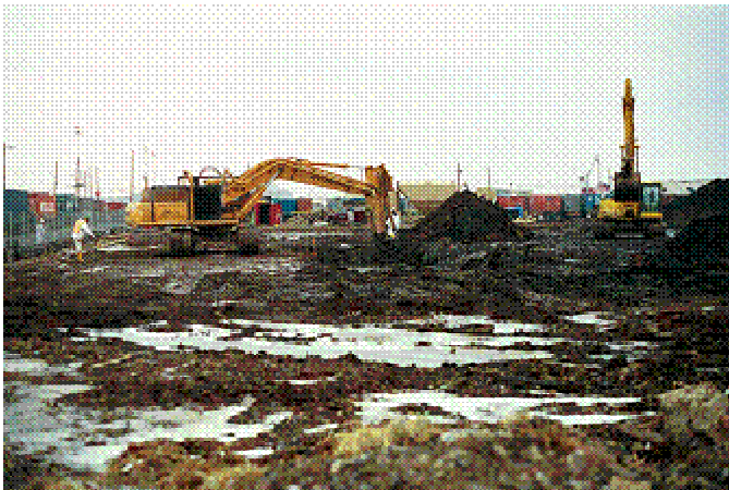
Figure 6.14: In-situ blender in use (Photograph courtesy of Colin Hills)
