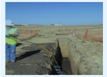
Use industrial or commercial waste to treat contaminants, such as waste cooking oil supplying carbon for a biogeochemical reactor. Travis Air Force Base, California
