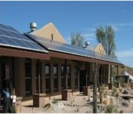
The solar canopy offsets approximately 45% of the energy consumed in the facility's administrative buildings while serving as a structure for rainwater harvesting.
