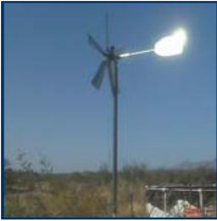
A windmill was initially used to generate mechanical energy for de-watering the perched zone below capped areas.
