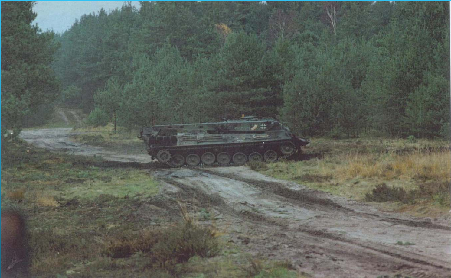
Building an access road to warfare agent pits
