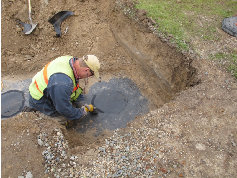
Photo 1. Roughing up surfaces of the high-density polyethylene liner.
