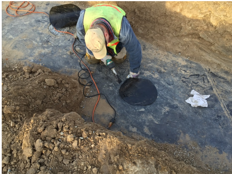
Photo 1. Welding process.
