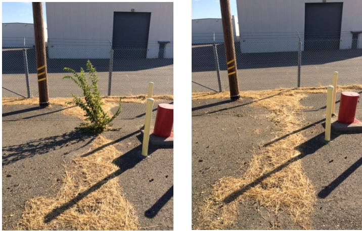
Finding 14-02 Tree Removal Along Northern Fence line
