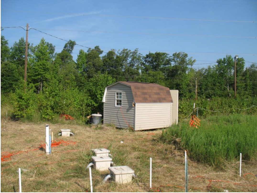
Figure 5-7 Shed housing the instrumentation
