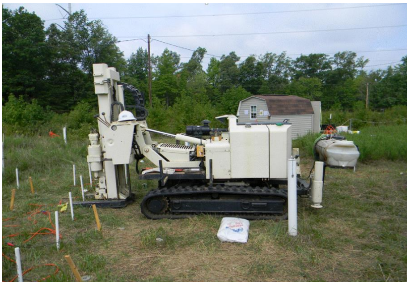
Figure 5-26 Direct push rig used for 2nd injection
