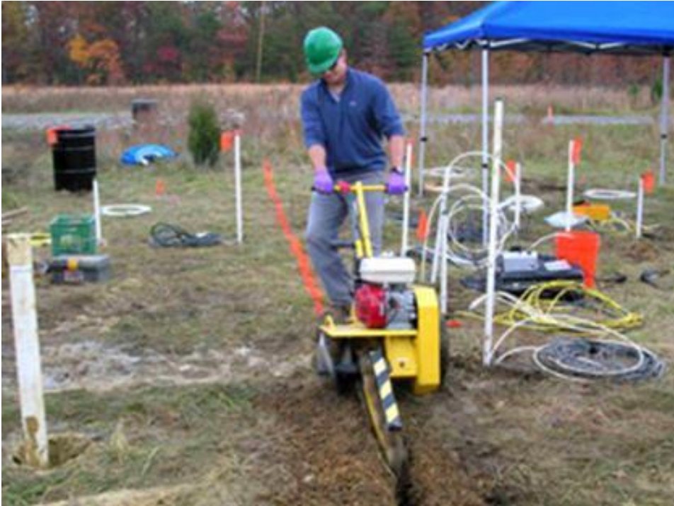
Figure 5-14 Installation of trenches for surface electrodes for the first injection experiment.
