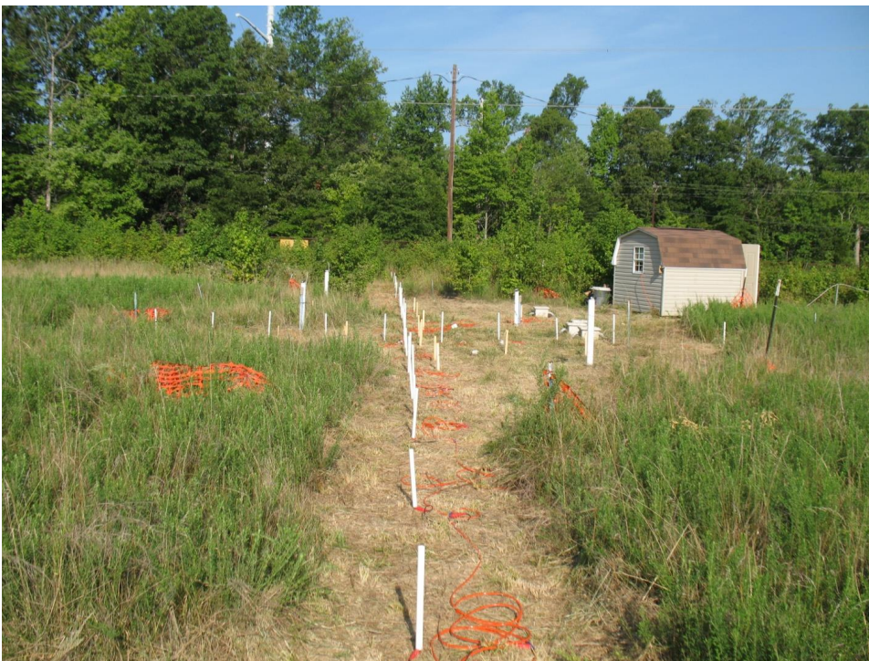
Figure 5-15 Surface array with temporarily installed electrodes for monitoring second injection experiment.
