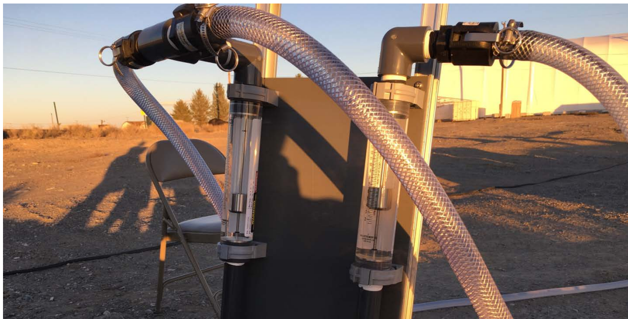
Figure 10. Inlet flow control during testing.
