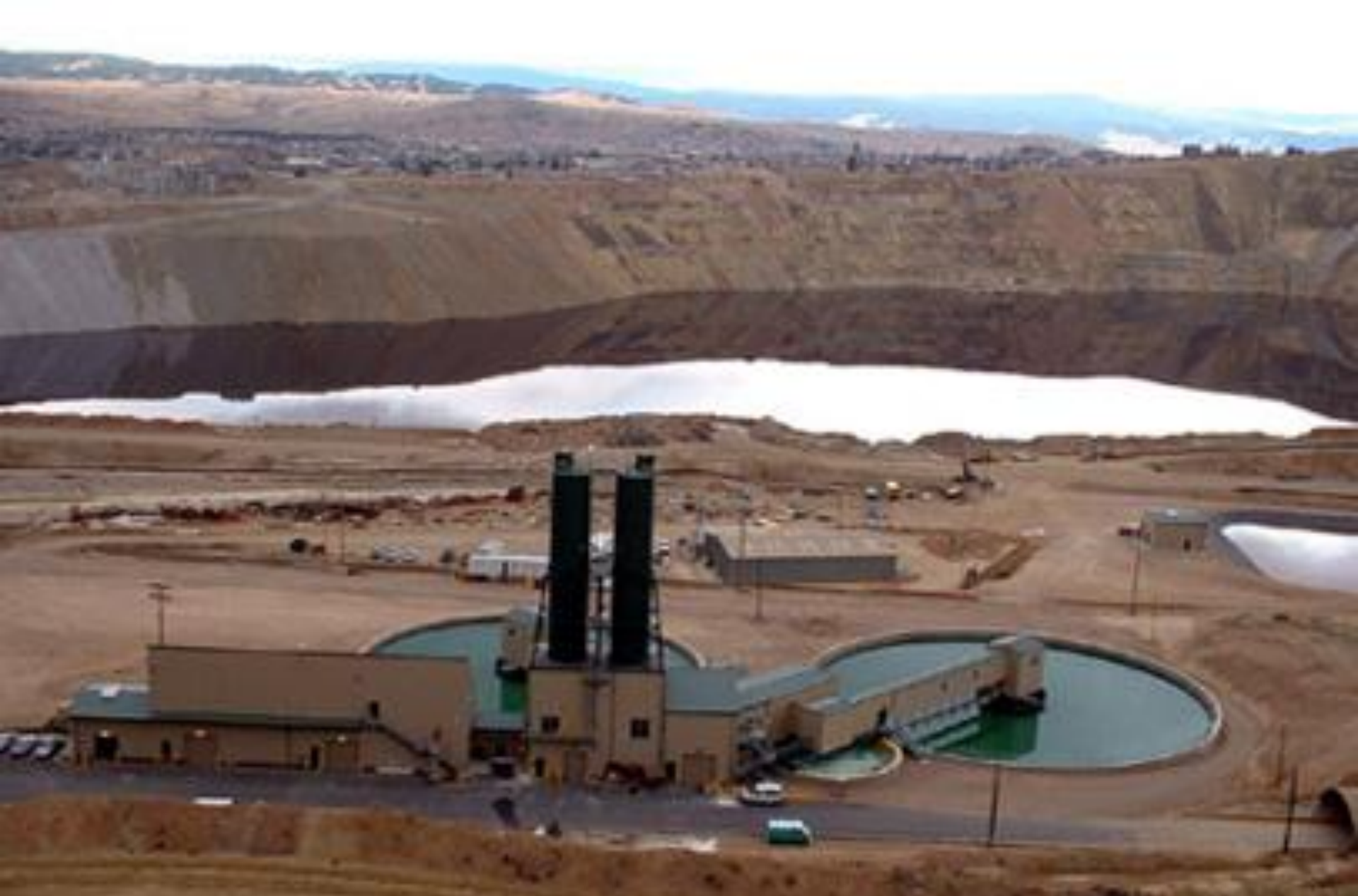
Horseshoe Bend Water Treatment Plant
