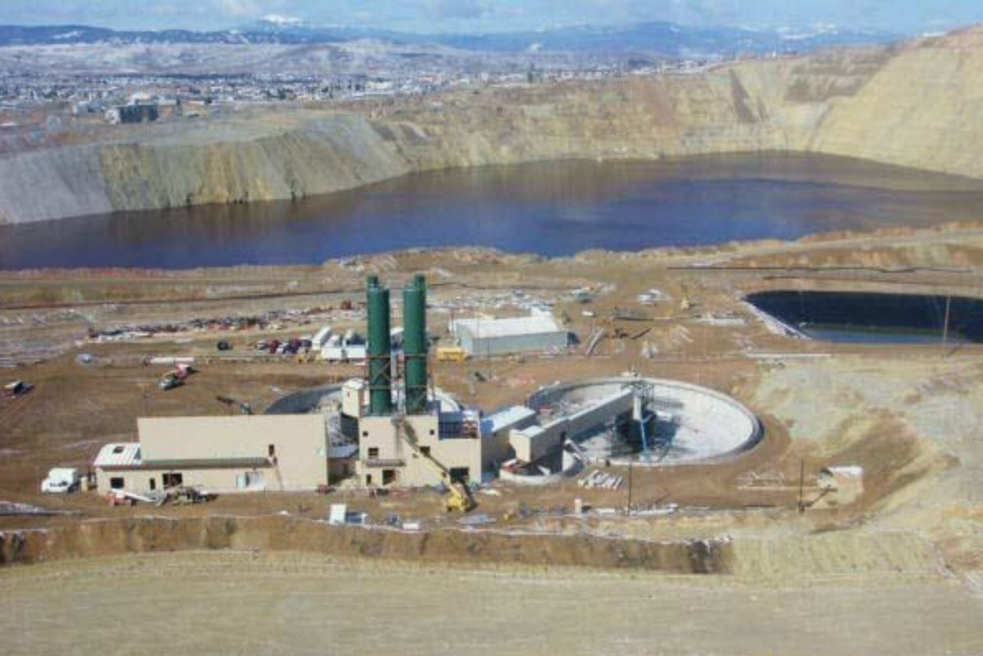
Horseshoe Bend Water Treatment Plant
