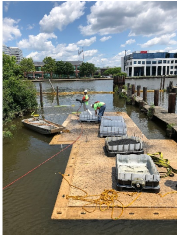
Application of inoculated SediMite™ to A-Street Ditch Segment 1 sediments.
