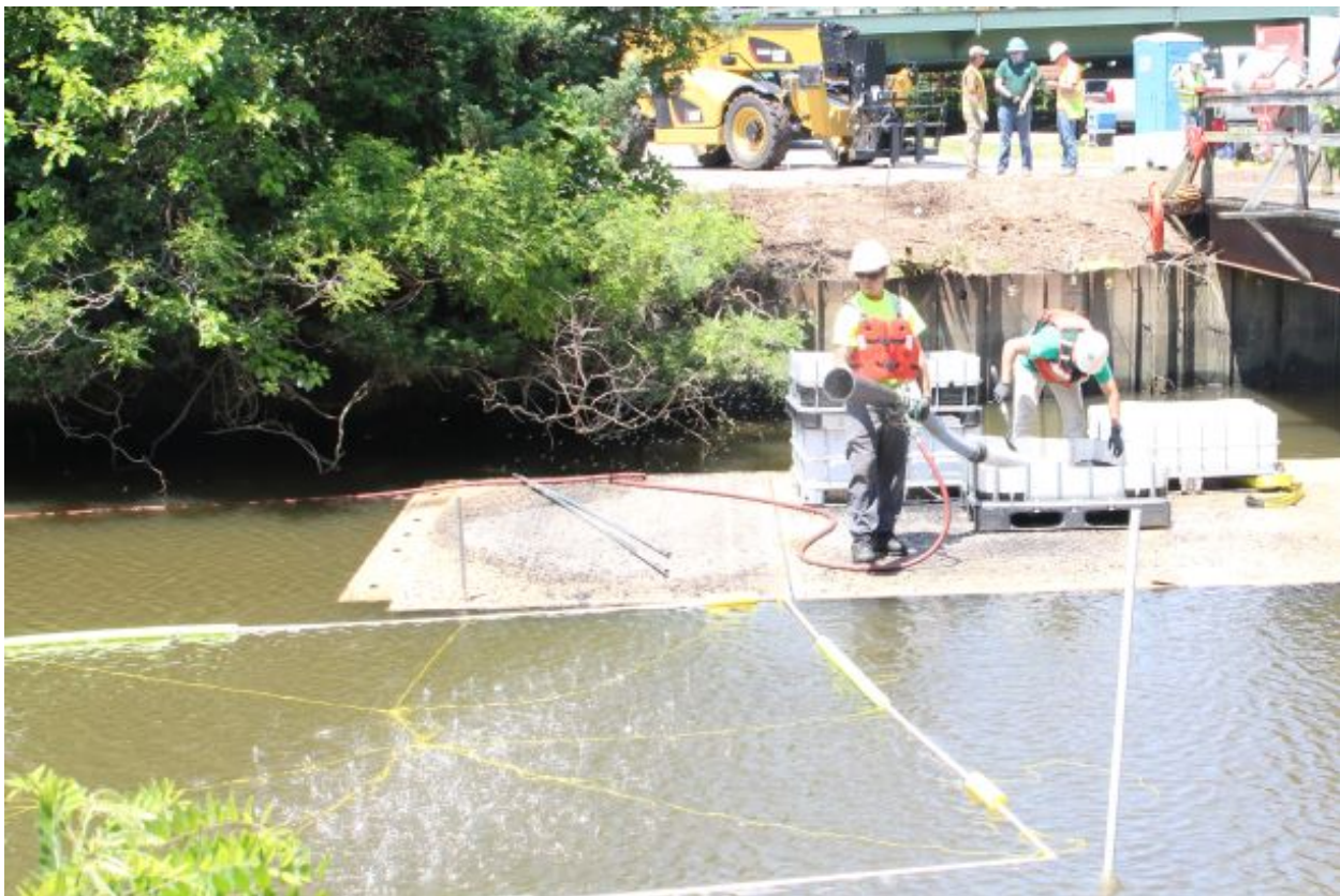
Figure 2b. Bioamended SediMite being applied to Segment 1 of A-Street Ditch.
