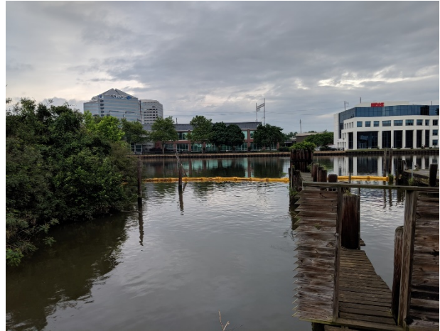
Turbidity curtain installed at mouth of ditch prior to SediMite™ application.
