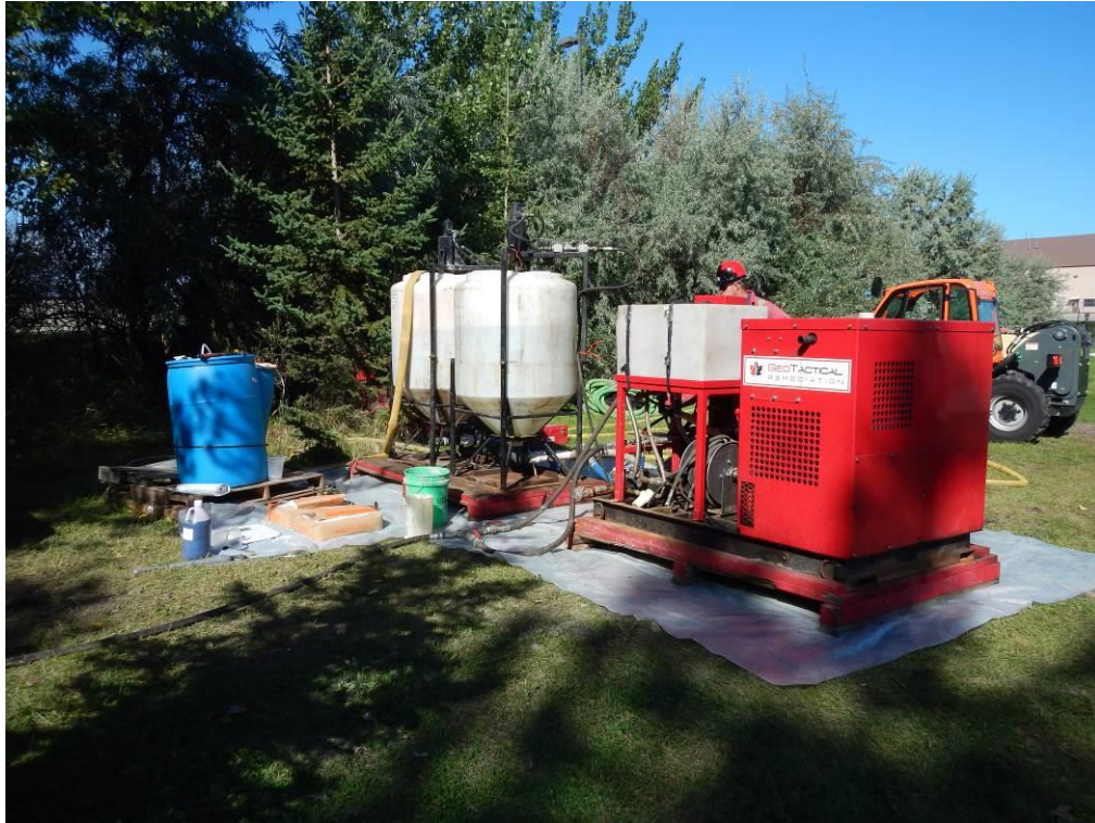
Photo 1 – EFI2000 Mixing and Pumping Unit with Ancillaries
