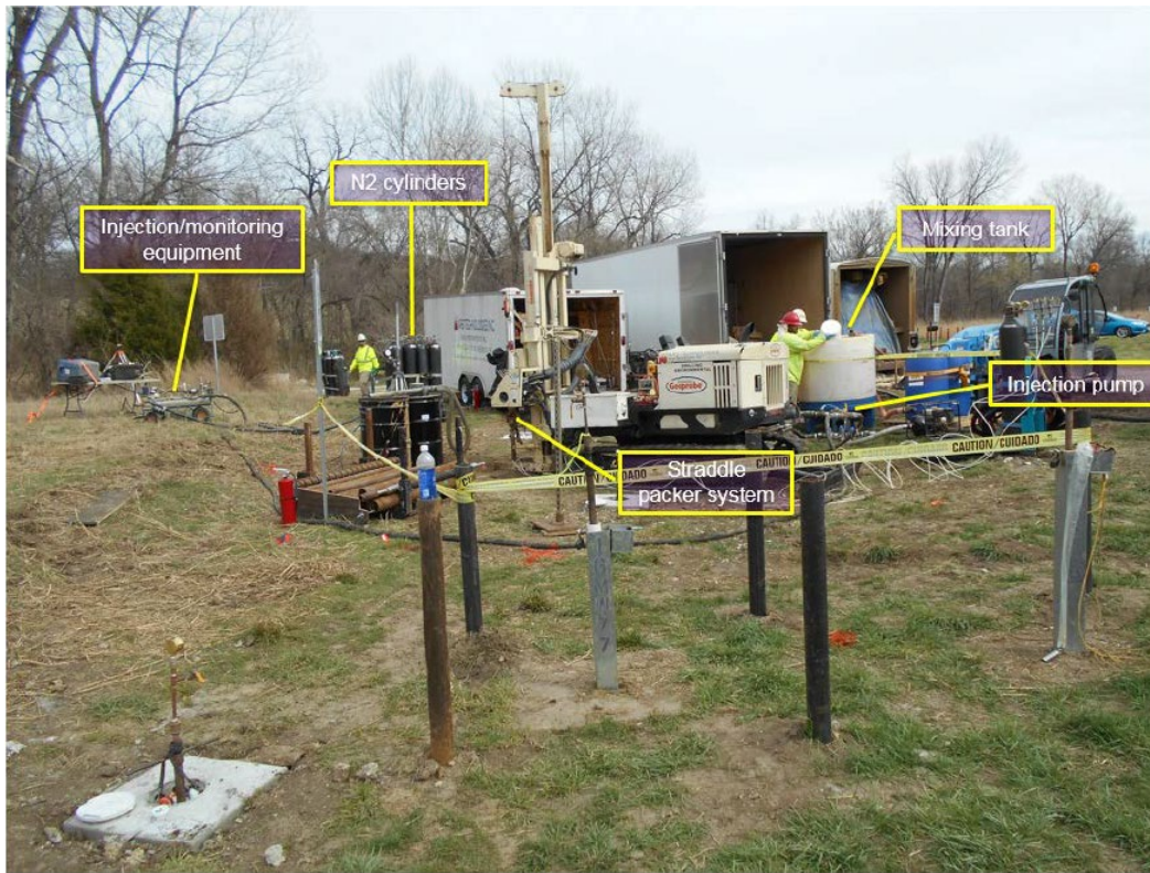
Figure 5.17. Aboveground Setup of Pneumatic Permeability Enhancement at LCAAP
