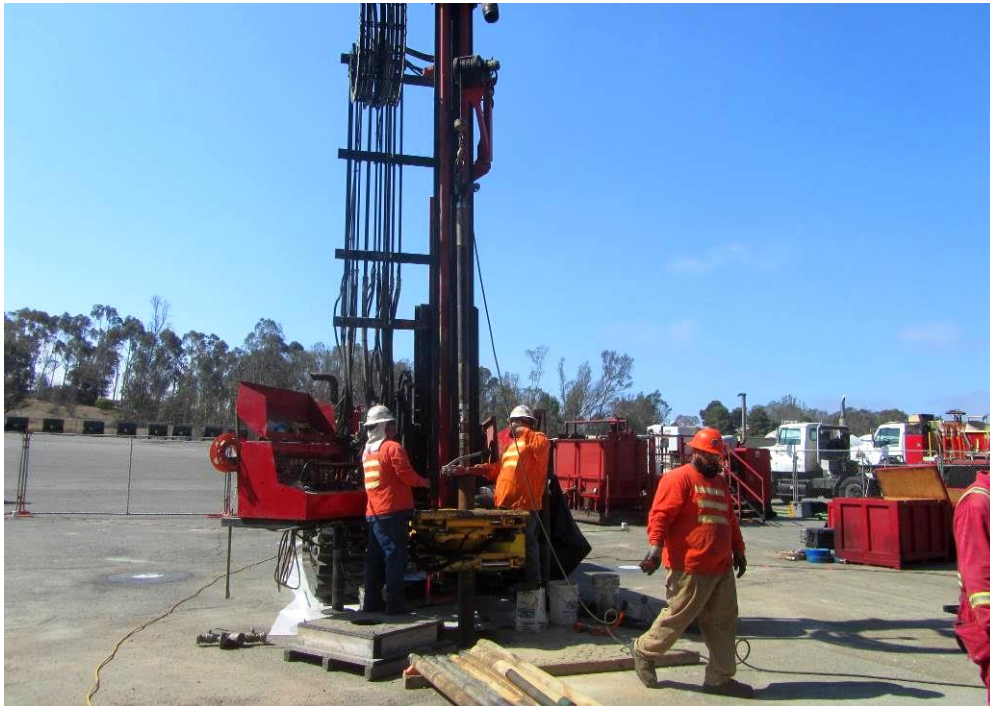
Photo 3 – Straddle Packer Assembly Being Lowered in HIW-01
