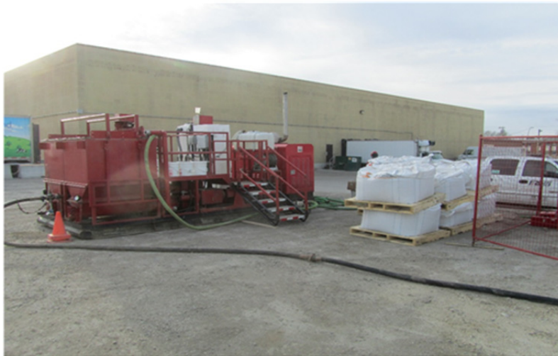
Figure 5.1: Typical Setup of the EF9300 Hydraulic Permeability Enhancement Unit
