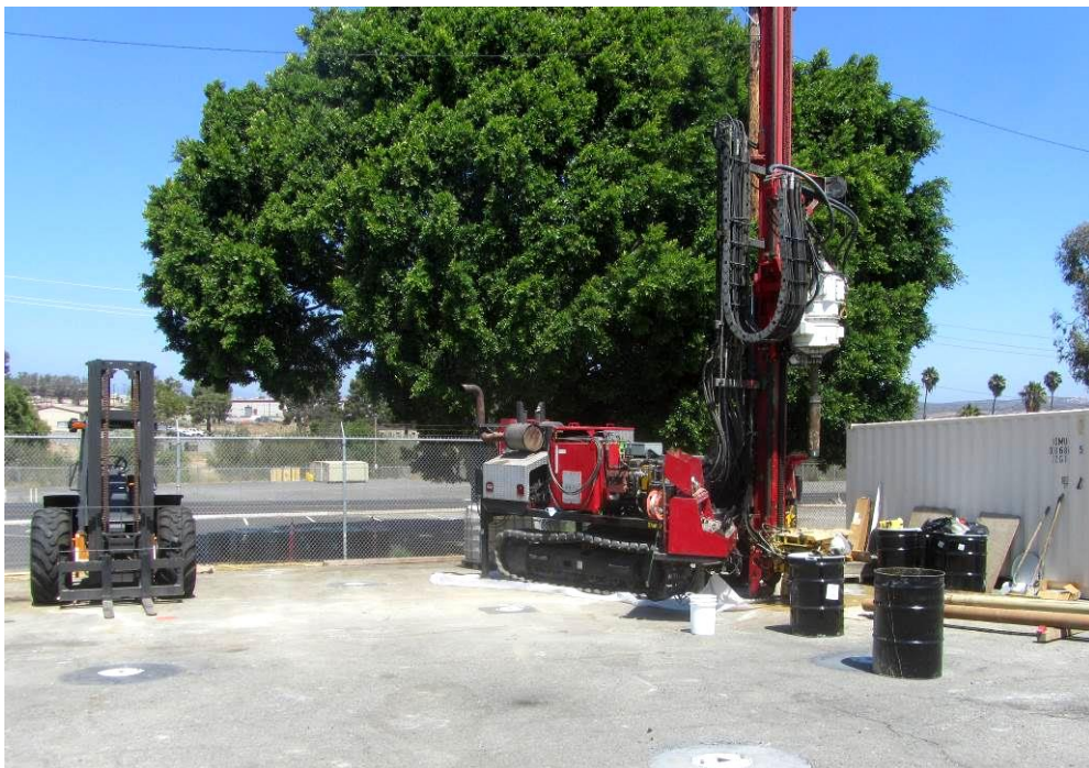
Photo 2 – Cascade's Track Mounted Sonic Drilling Rig
