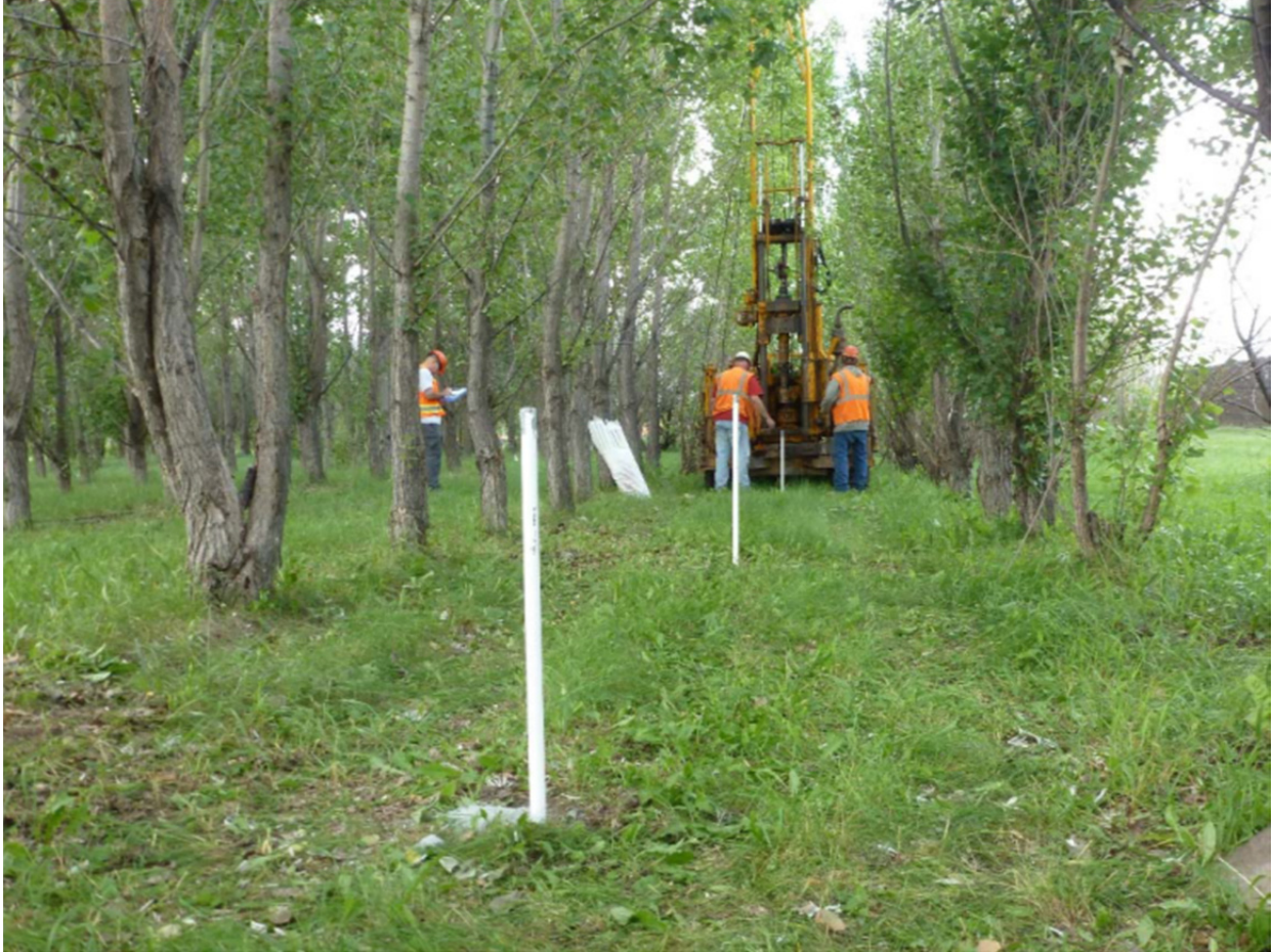
Figure 4.11: Temporary Injection Well Installation at the Grand Forks AFB Site TU504
