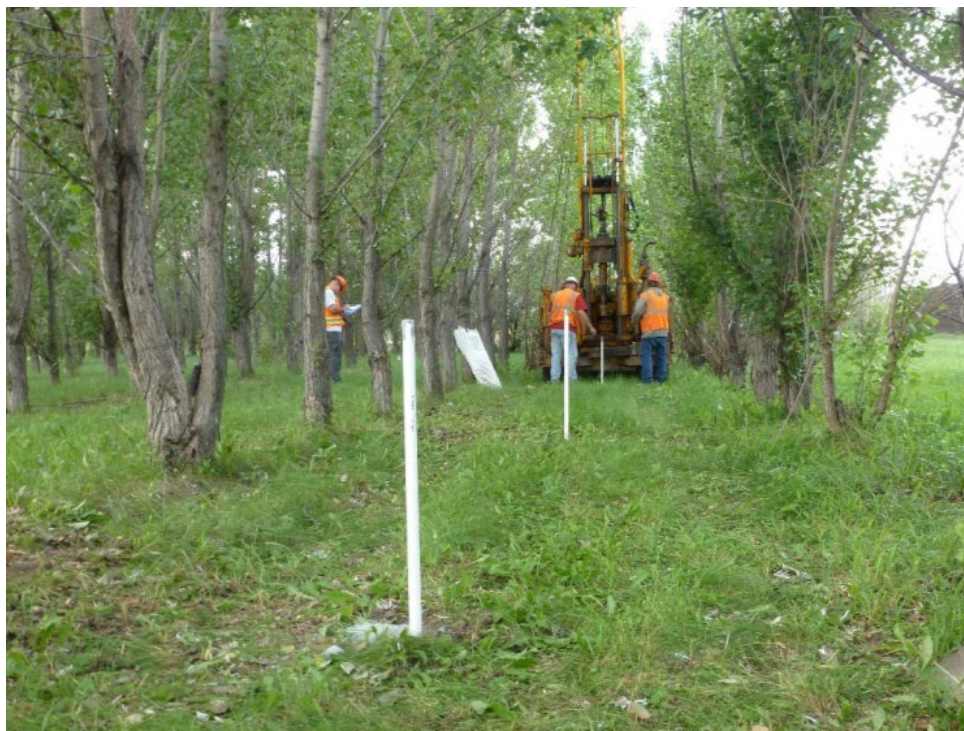
Figure 3.11. Temporary Injection Well Installation at the GFAFB Site TU504
