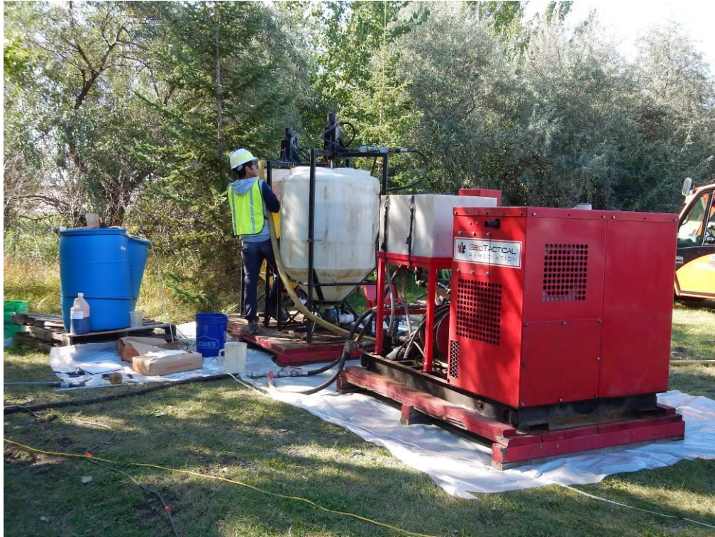
Photo 3 – Adding Potable Water to the Mixing Tank Prior to Adding LactOil®
