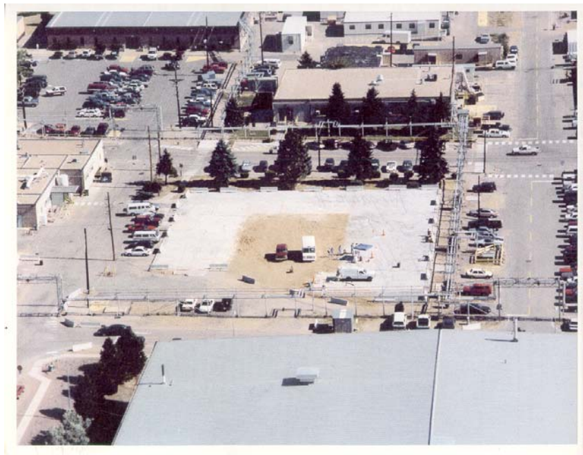
Figure 1. Under Building Contamination 123: the 'U' shaped concrete slab is located in the center of the photograph.
