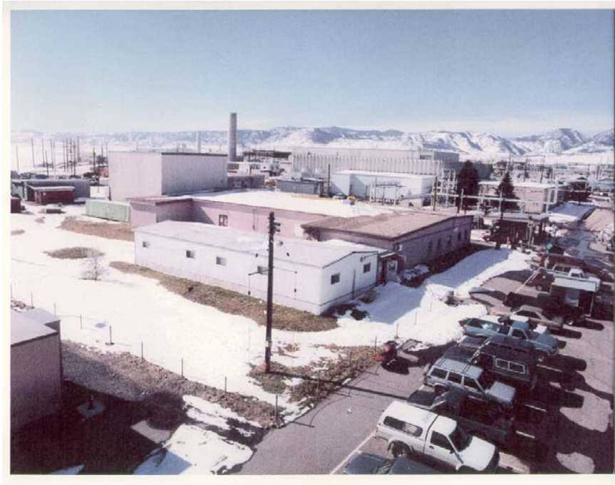
Figure 2. Building 886: building 886 is located behind the trailer.
