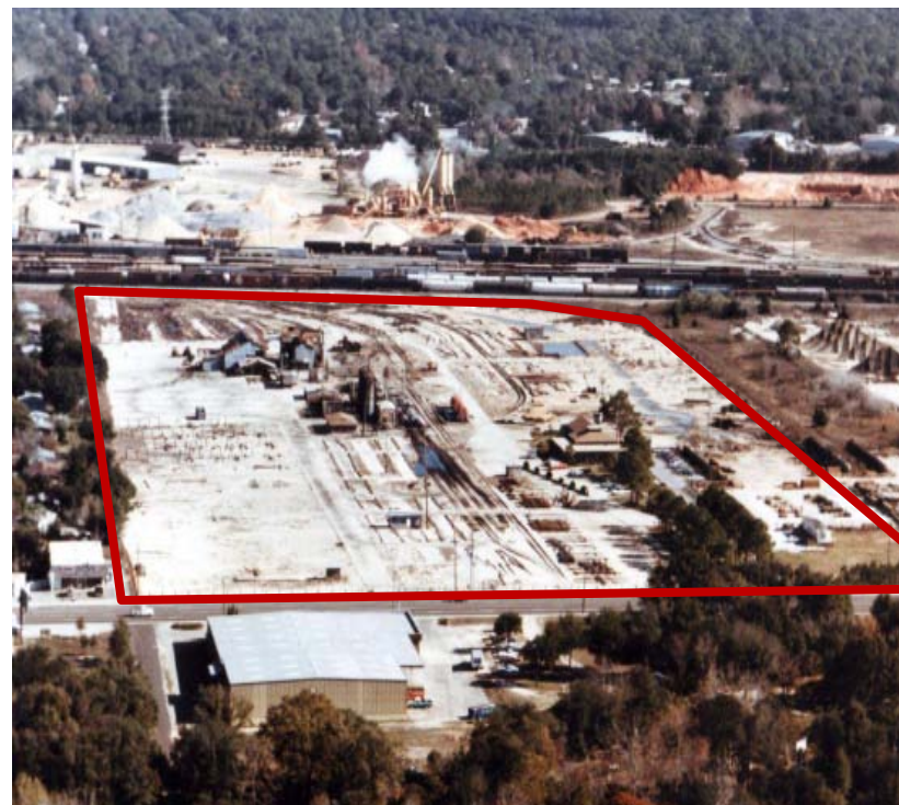
Active Wood Treating Plant circa 1975
