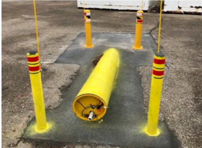
Figure 26. Wellhead Completion Entry (west) side well completion for the HRX Well.
