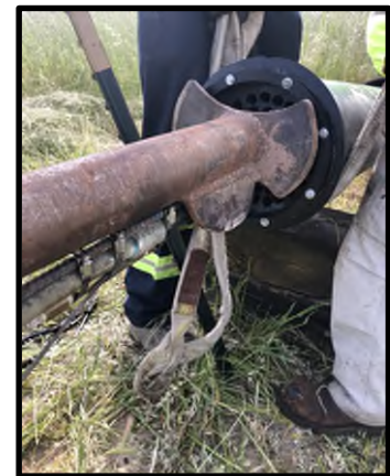
Figure 25. Monitoring Cartridge Installation
