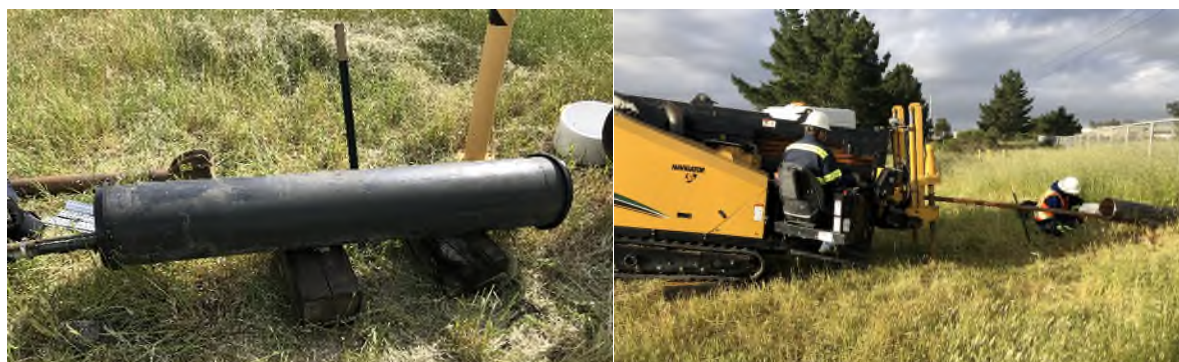
Figure 36. Installation of monitoring cartridges retrofitted with rubber seals
