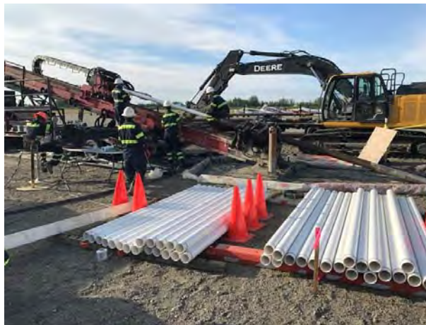
Drilling and well screen installation at Site ST005
