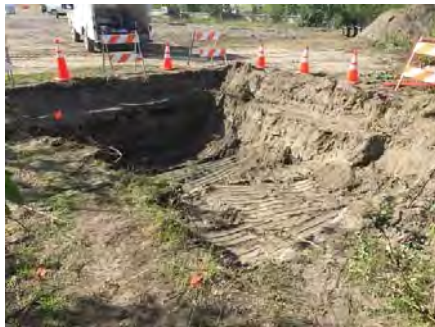
Excavation at Site SS017
