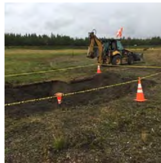
Excavation at Site CPL006 Area 3
