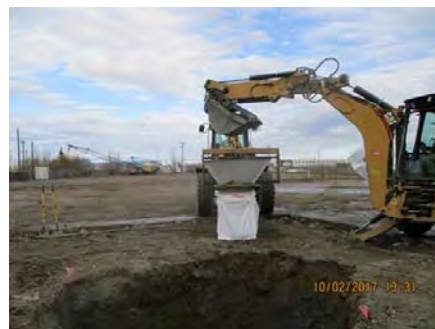
Excavation at Site SS014
