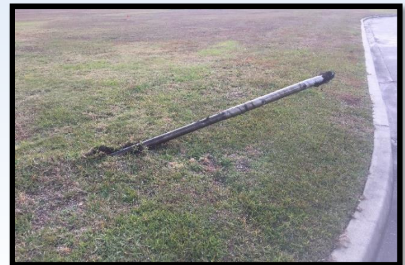
Drill Bit Exiting for Entry-Exit Well
