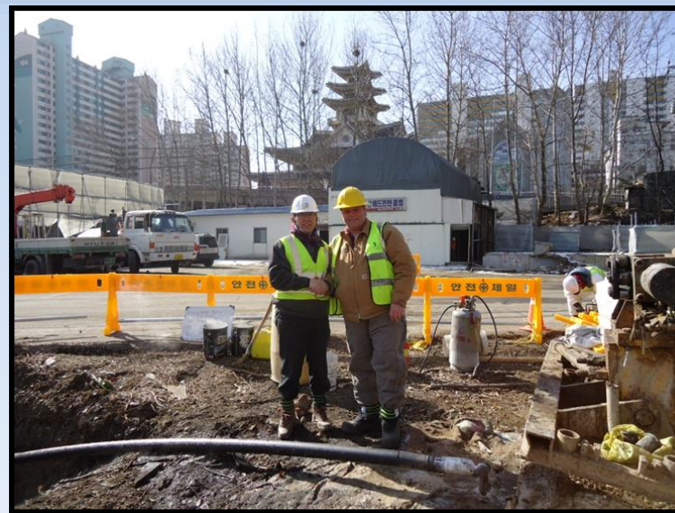
Installing first ever horizontal remediation wells (HRWs) in South Korea
