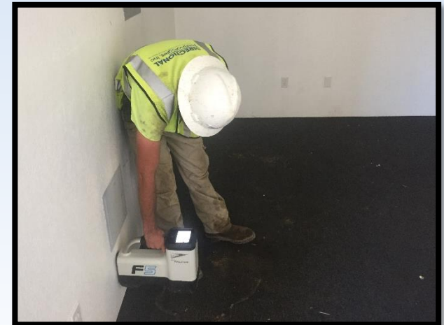
Real time tracking beneath building slab.
